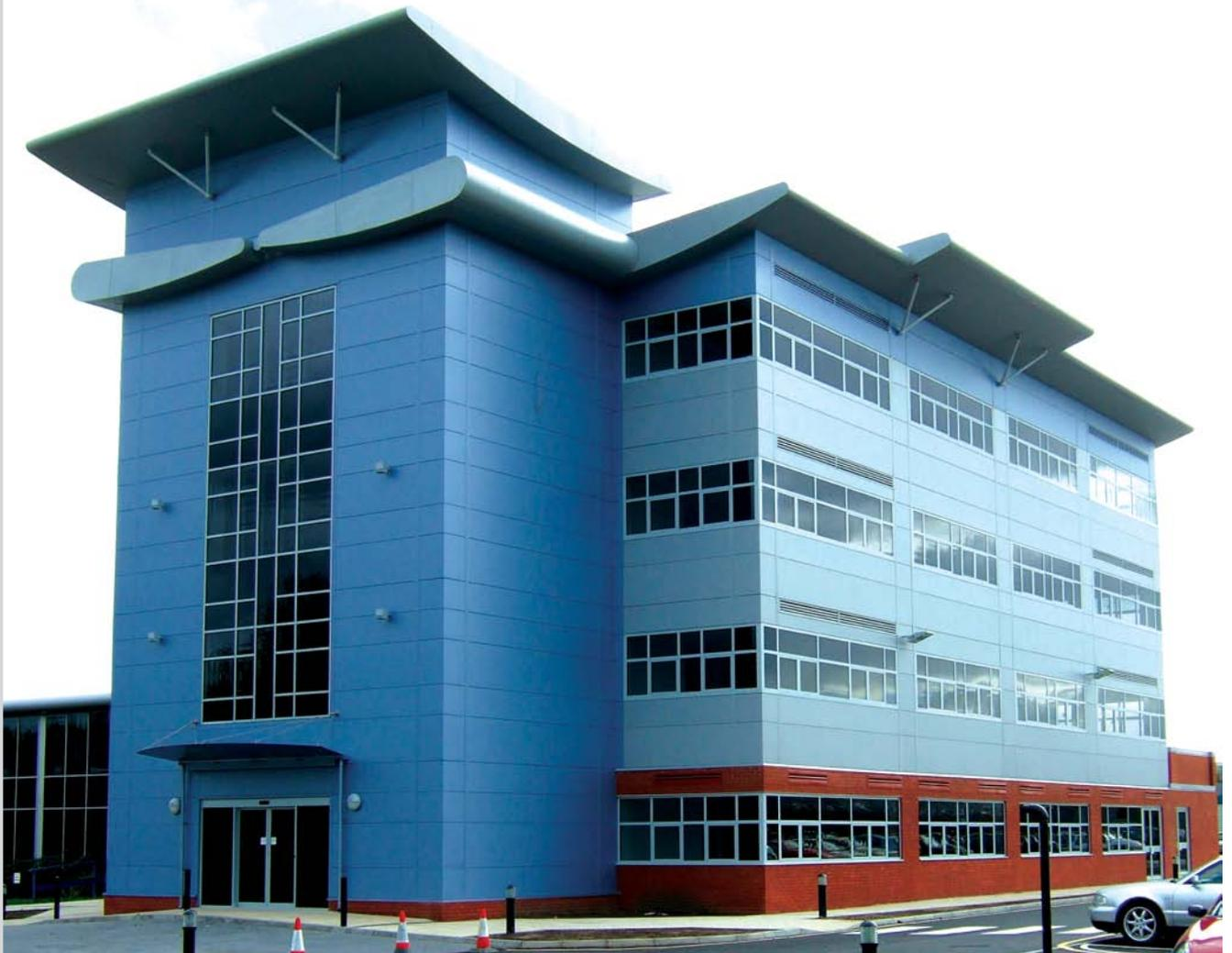
Phoenix Place office development located in Basildon, Essex tenants include the local NHS Primary Health Care Trust. Dovetail Architects designed the building, selecting W.A. Hills as the contractor, with Comar approved fabricator Anglia Fixing Limited to complete the glazed element of the facade.
